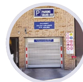
Parking couvert Grand-Rue 30, Grand-Rue L-4575 Differdange
